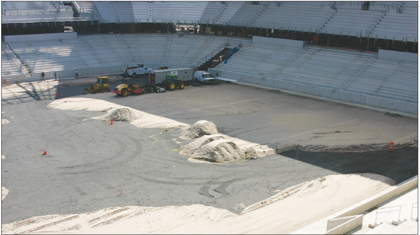
Red Bull Arena field construction. Credit: Z. Holm.
