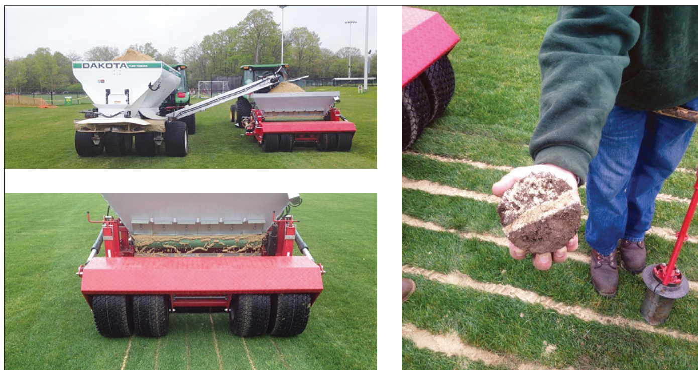
Sand-slit drainage system installation. Credit: B. Polimer.
