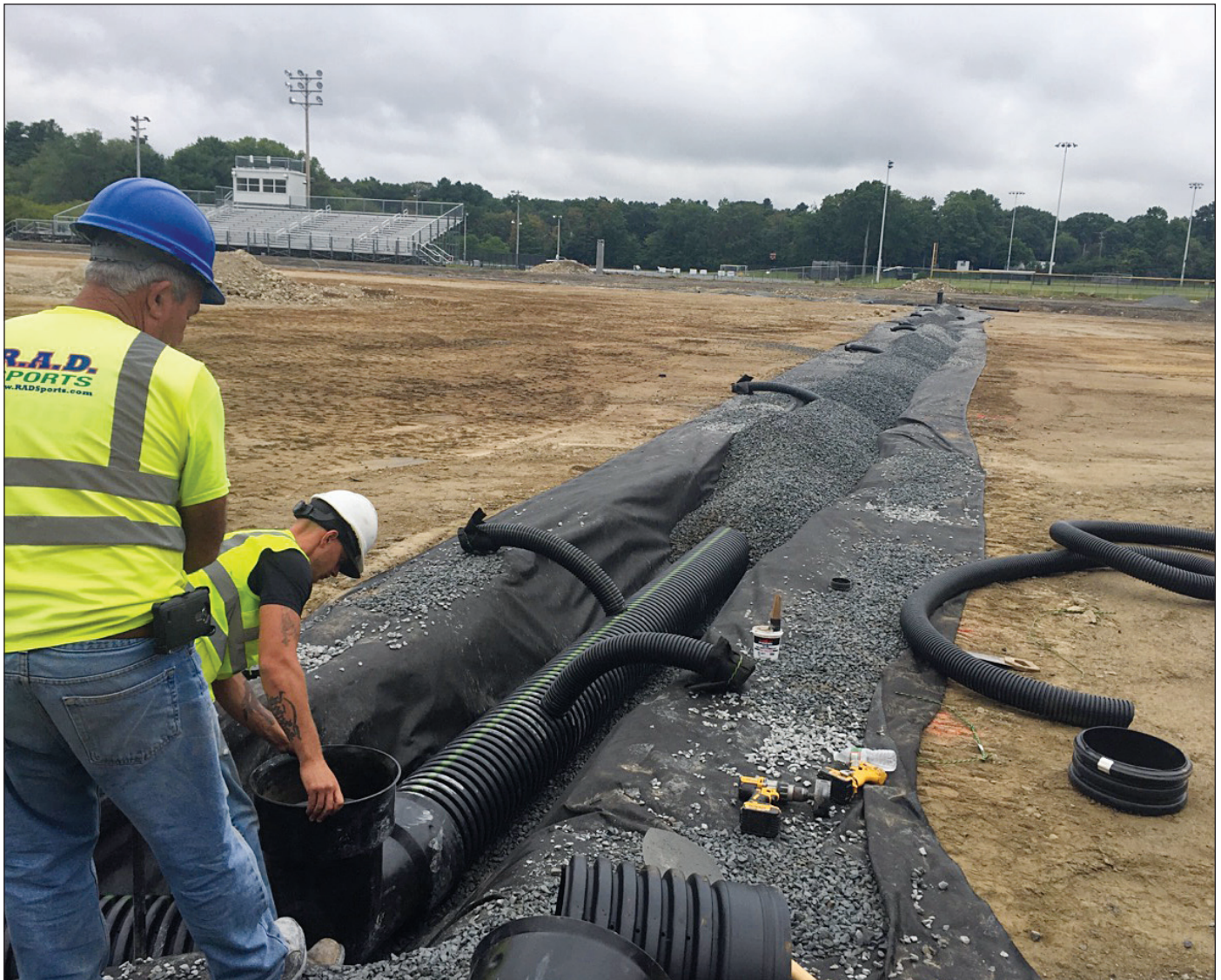
Installing curb drainage. Credit: B. Polimer.
