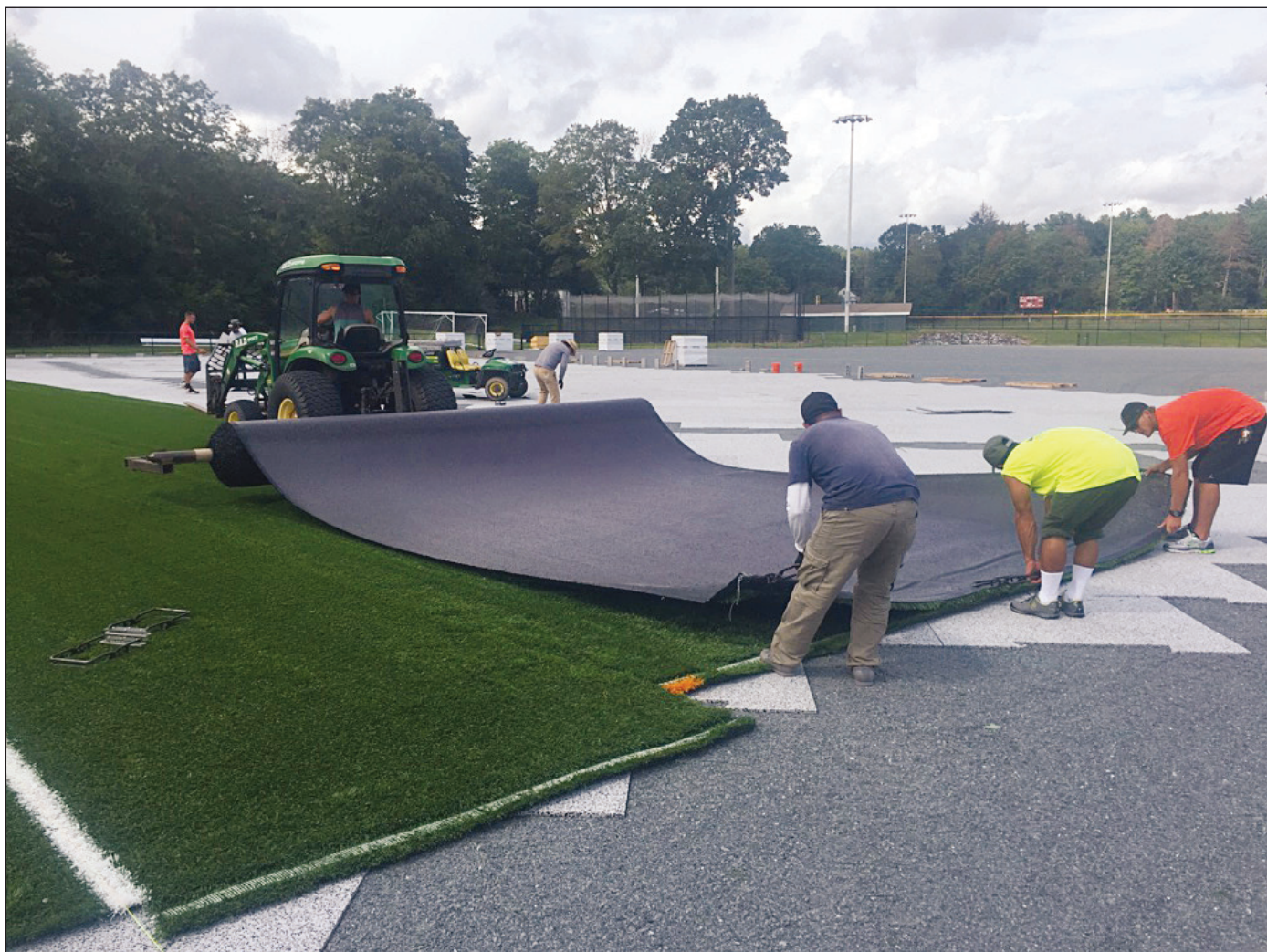
Synthetic turf installation. Credit: B. Polimer.
